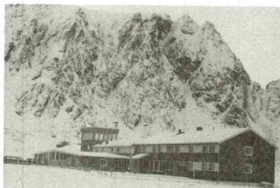
RANGE CONTROL CENTRE
